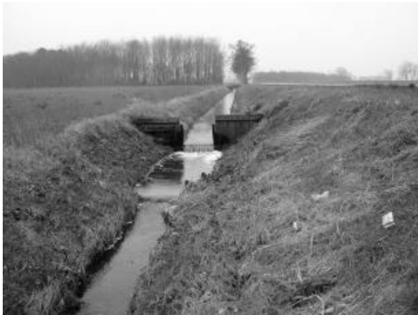
A weir with movable crest to remove excess water in winter (left) and retain water in summer (right) at Chaam, province North Brabant, the Netherlands (Pictures courtesy of Jan Hoevenaar)
